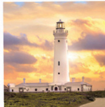
Lighthouse - Cape St Francis
