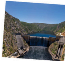
Kouga Dam - Patensie
